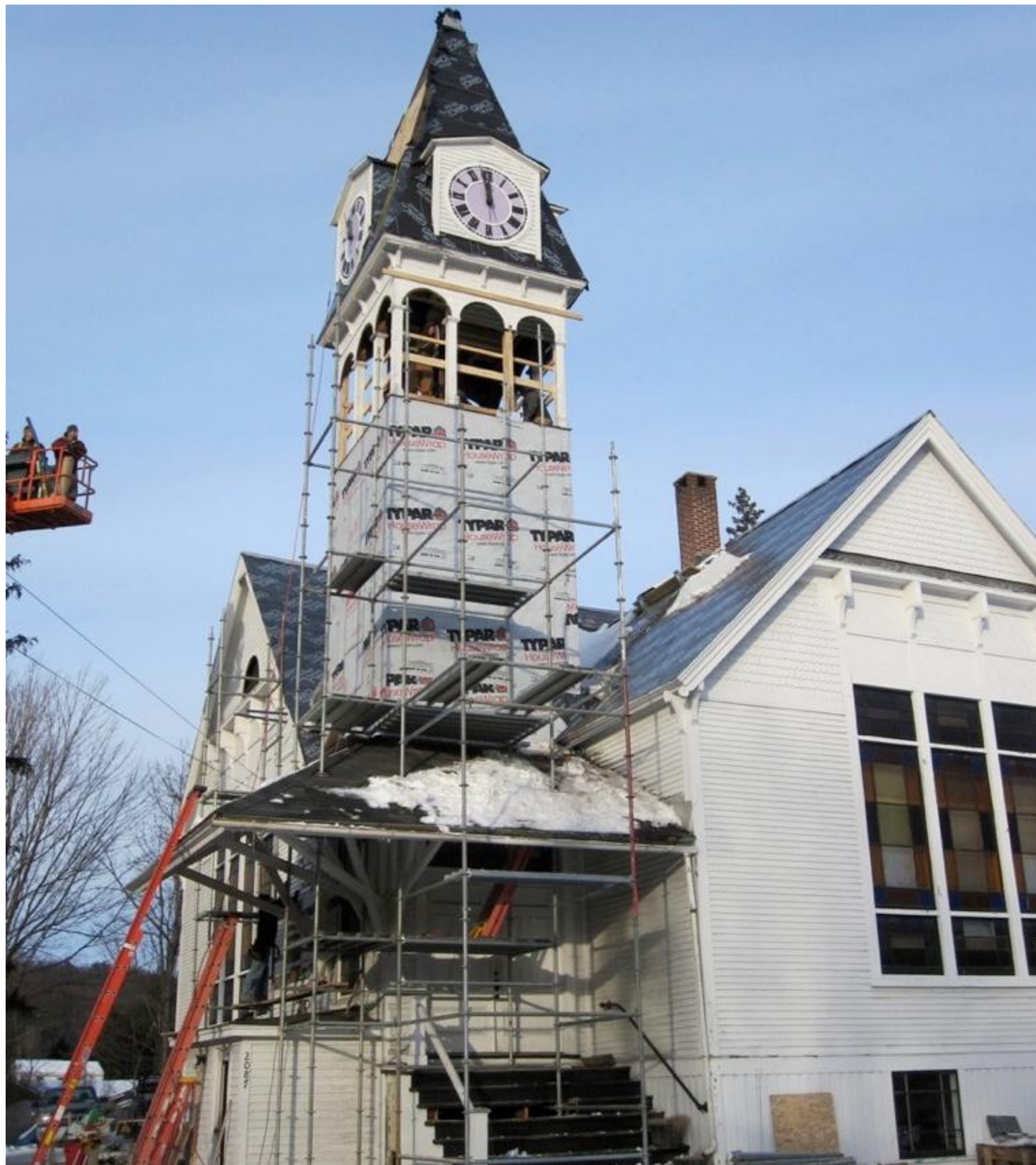
Brian Gardner Carpentry of Etna, N.H, completed the steeple restoration during the winter of 2009–2010. The original slate roof pattern was matched and restored by Hayward Roofing of Chelsea, Vt.
